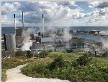
Green roof with plants around
