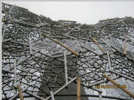
Mount Shidare closeup of roof structure (photo © Olga Popovic Larsen)
