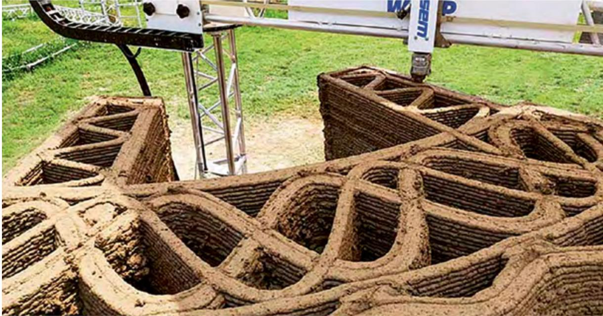
Figure 2.3.7. WASP is using its Crane 3D printer to build TECLA | Image via WASP (3dNatives, 2020).
